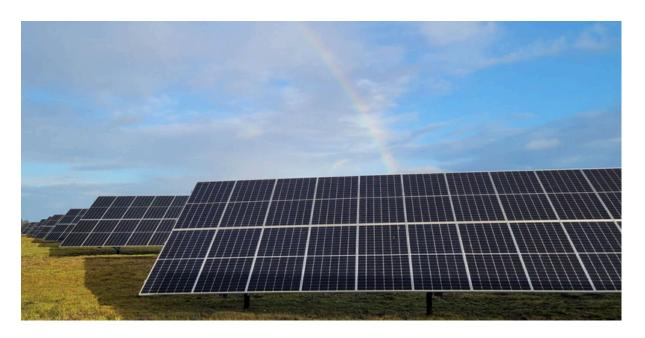
Hedgehog Technologies partnered with the Haida Nation to design and install a 2MW solar array and battery to form a microgrid, with expansion potential to 4MW, prioritizing community ownership, management, and training.
